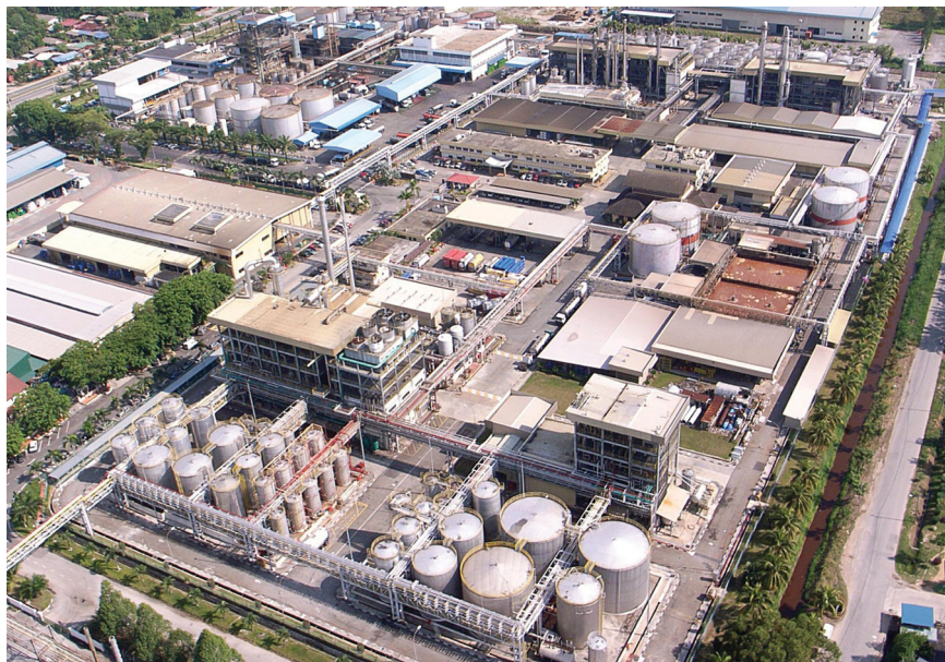
Emery Oleochemicals plant in Teluk Panglima Garang, Malaysia
